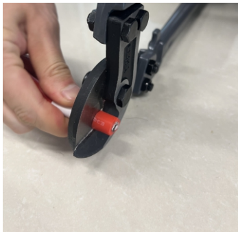
Cut the insulation of power cable gently
